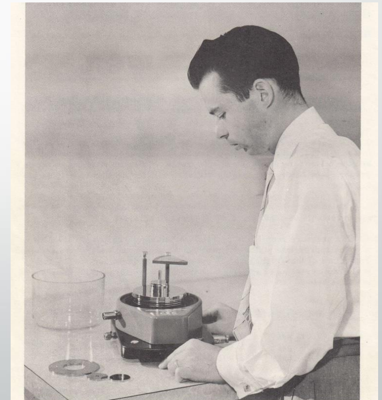
LEVELING THE 6-201-0001 PRIMARY PRESSURE STANDARD
